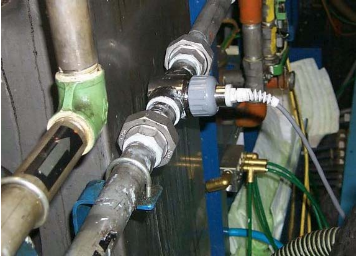
PR-111 Probe in horizontal pipe installation
